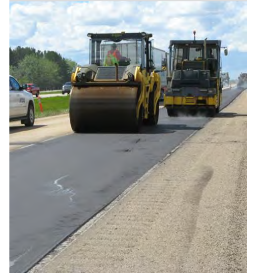
Highway 16 high strain crack relief interlayer trial project
